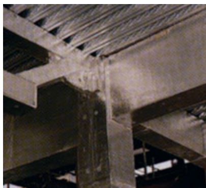
BeamClad A/F With Class 'O' reinforced aluminium foil, factory-applied to the outer face.
