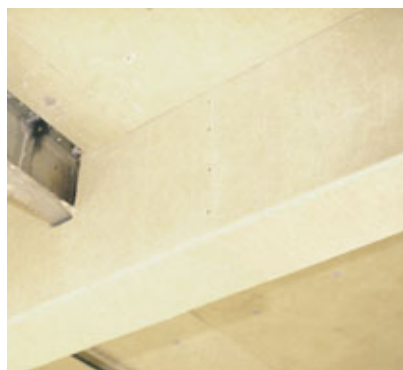
BeamClad T With a white glass tissue factory-applied to the outer face.
