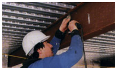
Fixing stud welded pins
